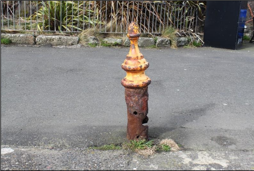
Figure 10a: Cast Iron Bollard, SW Corner of Basin A, S End of West Pier B4
