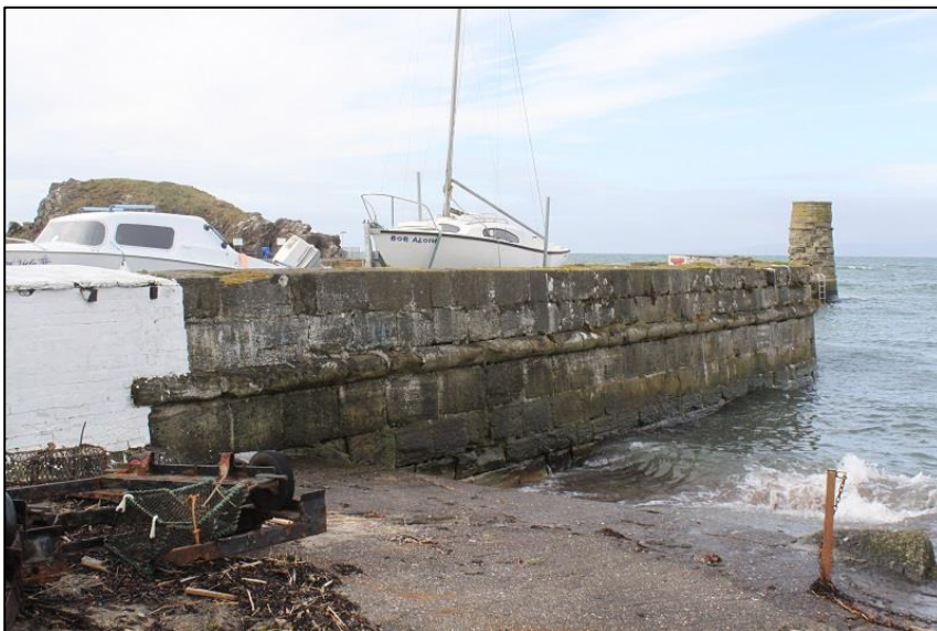
Figure 8c: NE face of North Pier B1
