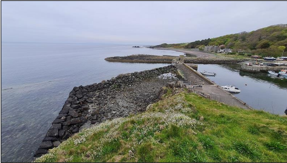
Figure 8a: West Wall B4 and breakwater E in Wider Context
