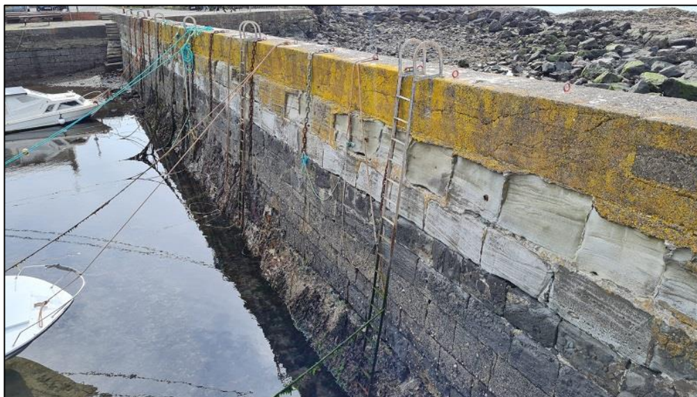
Figure 6c: Internal Face of Quay Wall B4 Fully Exposed at Low Tide
