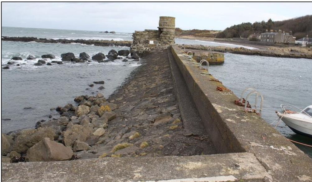
Figure 7c: View Along West Wall B4 , Showing Line of Raised Walkway
