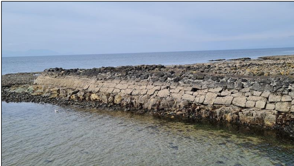
Figure 11b: Detail of W End, North Breakwater D , Showing Variation in Masonry
