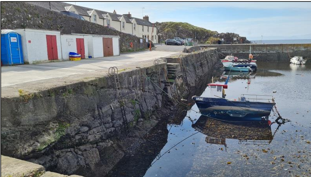
Figure 9b: Current Access Arrangements at South Wall B3
