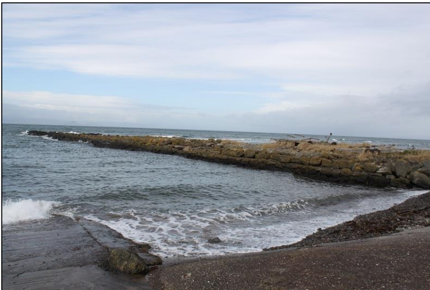
Figure 10c: General View of North Breakwater D
