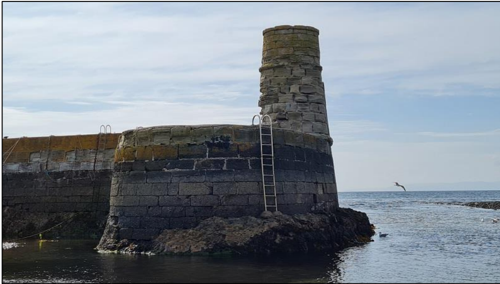
Figure 7a: N Terminal of West Wall B4
