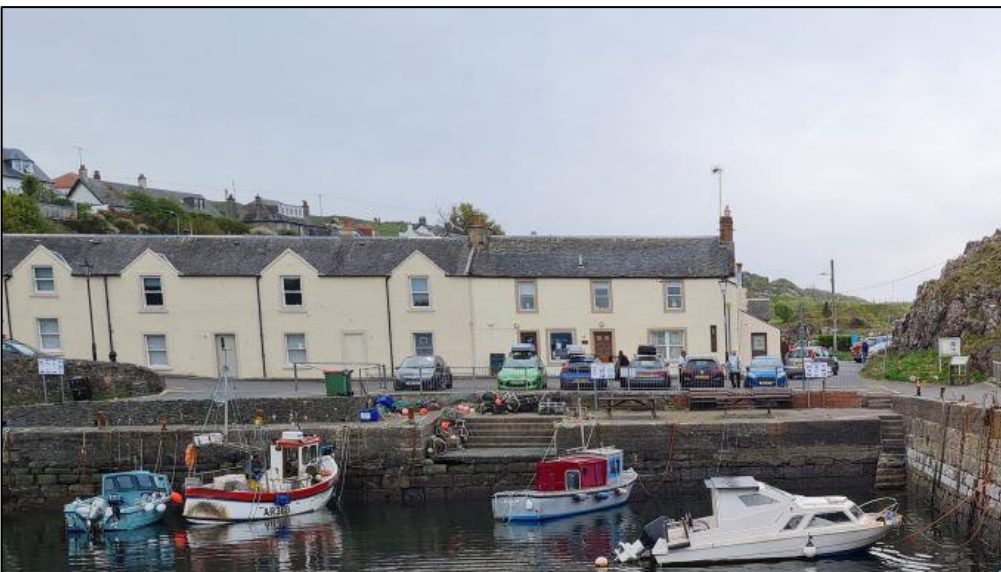
Figure 9c: Lowered section of South Wall B3
