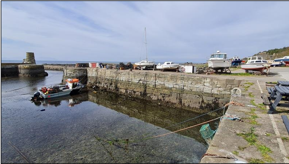
Figure 7b: Inner Face of North Wall B1
