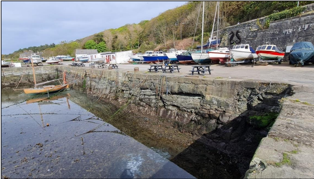
Figure 6a: Outcrop & Revetment Walling in E Wall B2 of Harbour
