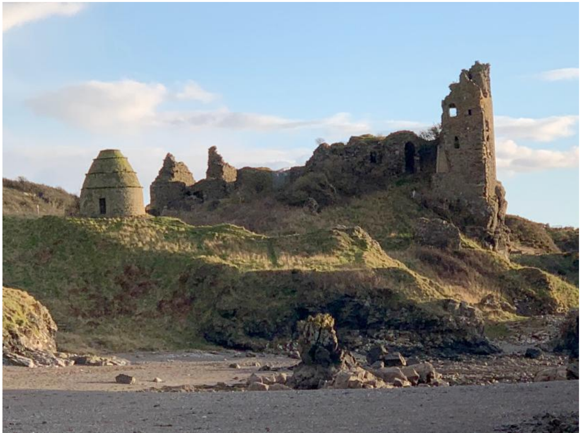
East elevation. Substantial fragments of structure have fallen on the north side and lie on the grass bank between the Castle and Dovecote
