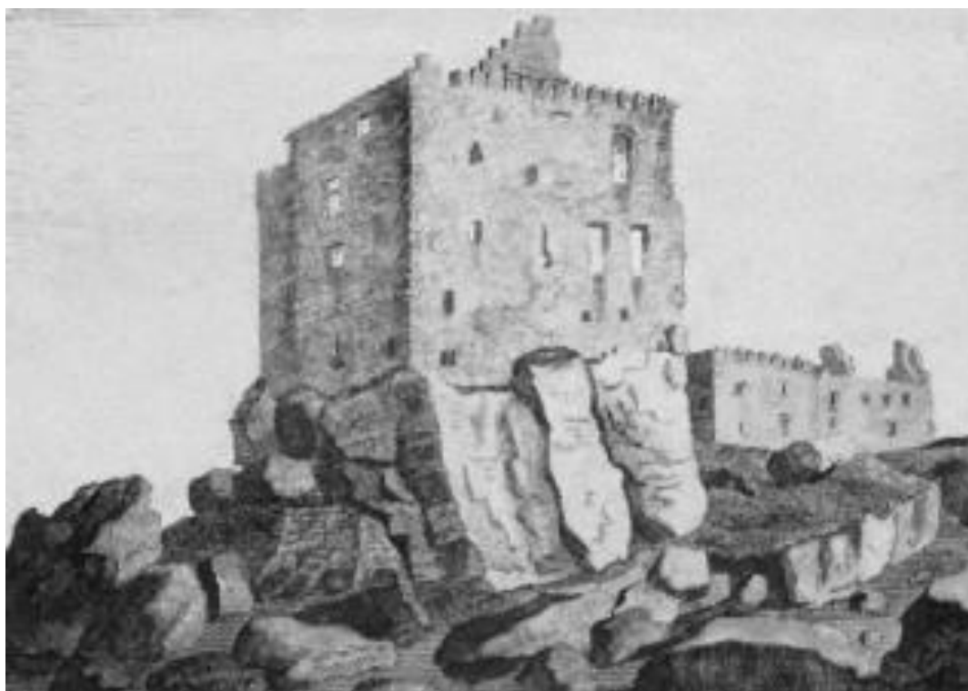
The view from the beach below the castle cliff illustrates the scale of the main tower structure before later sections have collapsed
