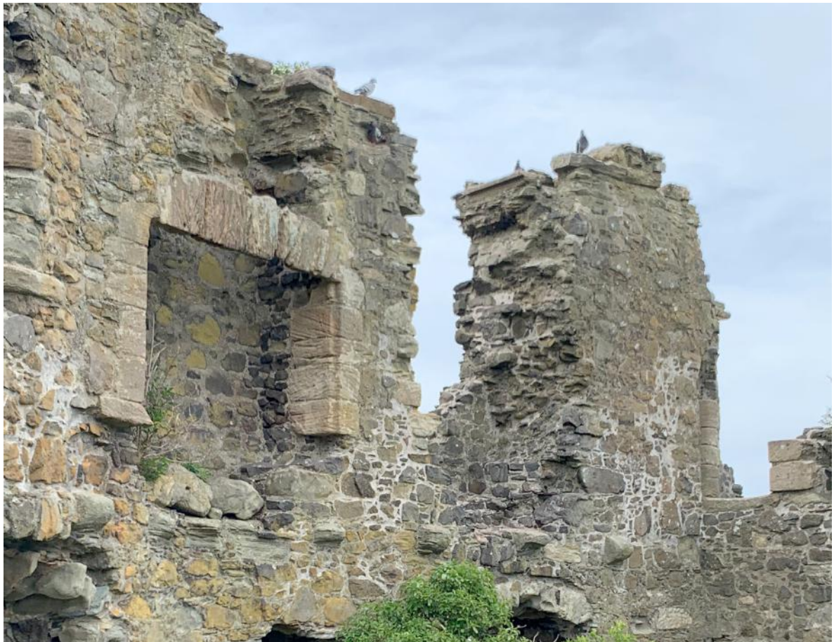
Loose stones at high level and erosion of mortar and stone of tower west wall and fireplace
