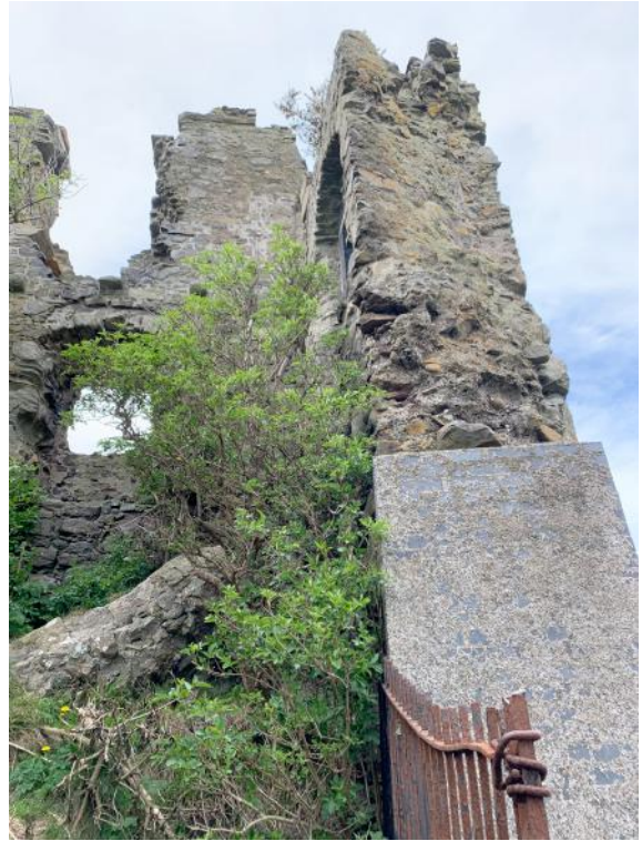
Vegetation growing up West elevation and trees rooting in high level mortar joints
