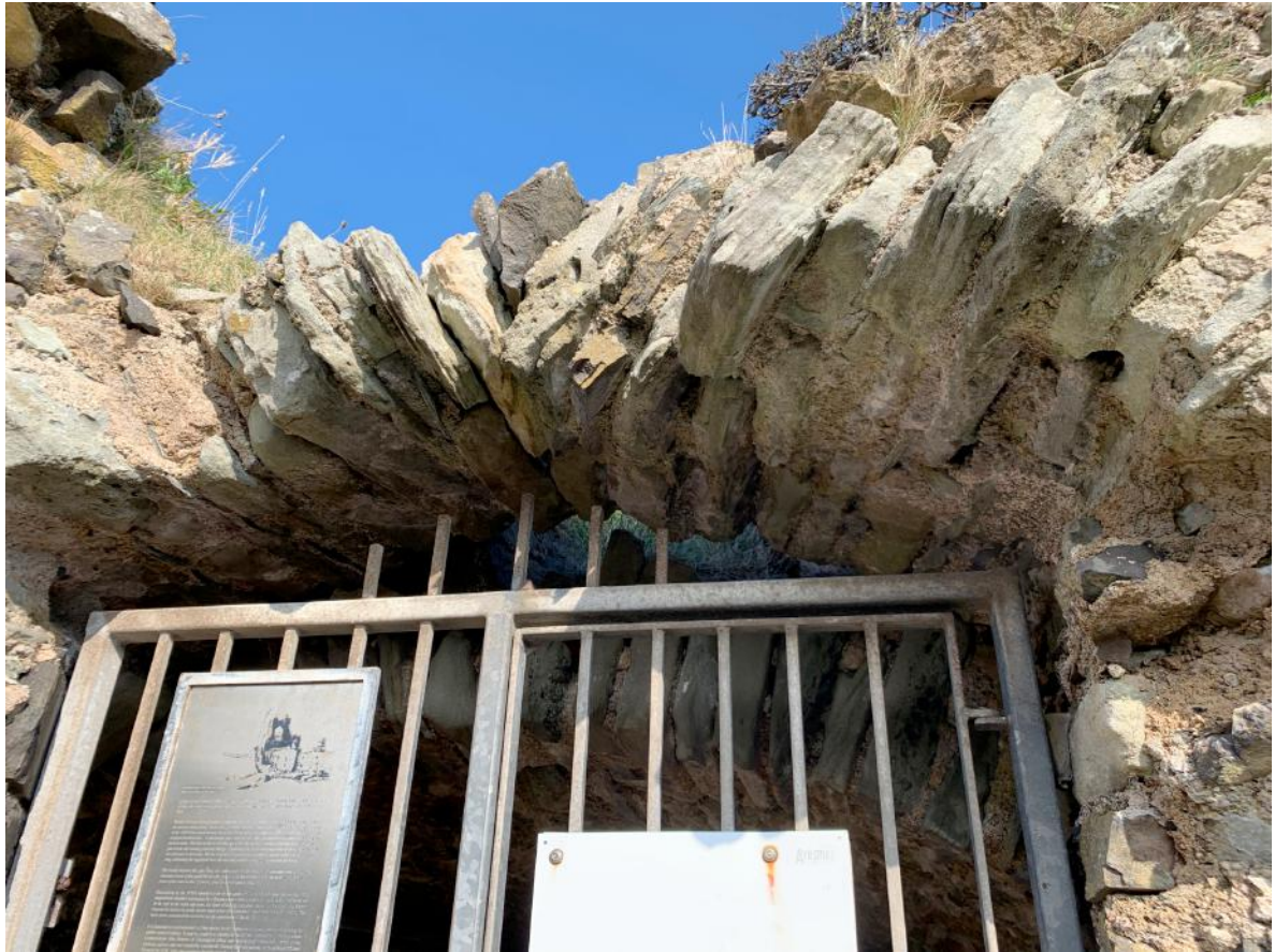
Loss and erosion of mortar in arch of gated access to tower
