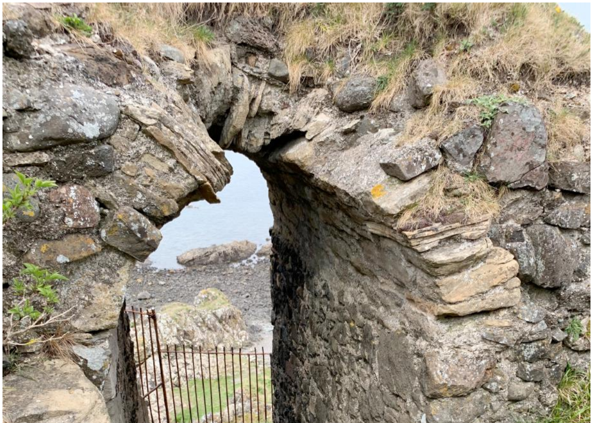
Loss and erosion of mortar in arch of gated access to tower
