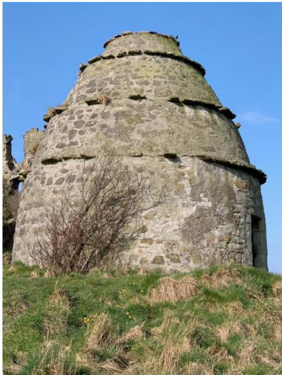
Dovecote masonry condition is sound, with minor vegetation growth at high level
