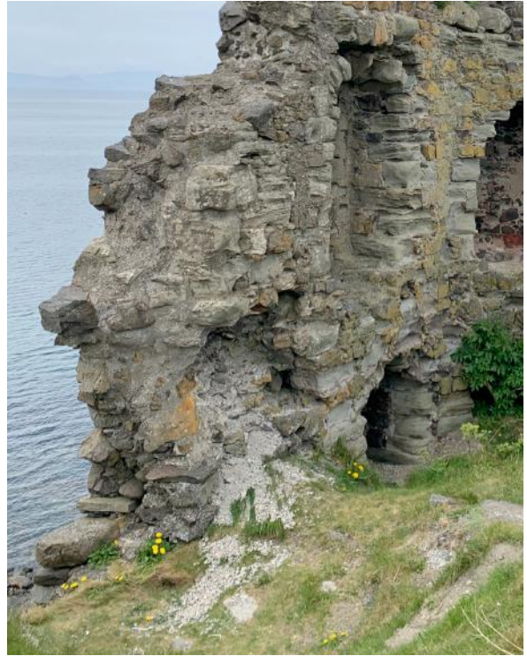
west elevation tower loose stone low level
