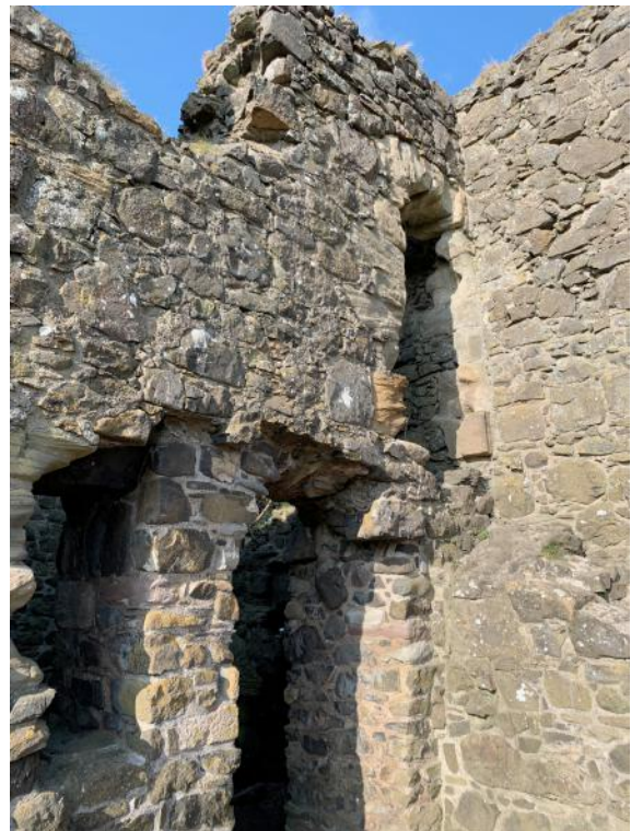
Some loose stones fallen out of tower NW corner and chimneys of South building
