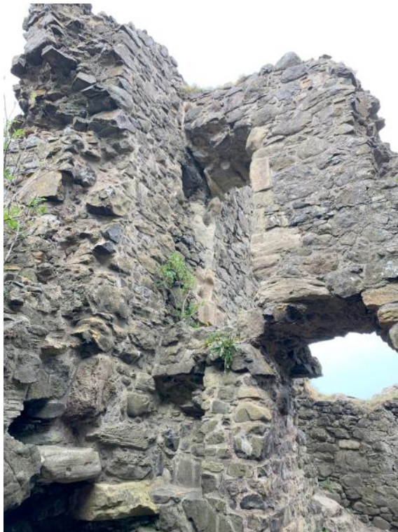
Some loose stones fallen out of tower NW corner and chimneys of South building
