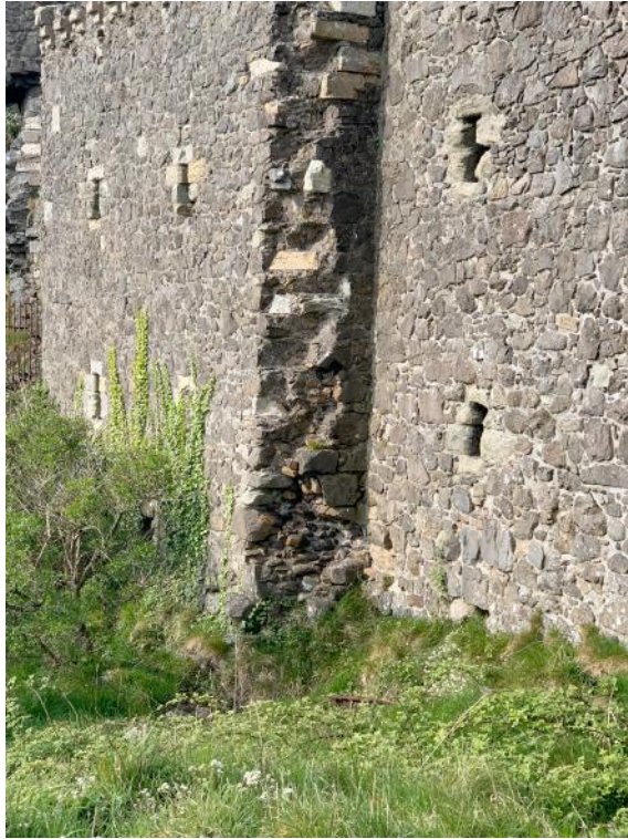
Vegetation growing up West elevation and trees rooting in high level mortar joints
