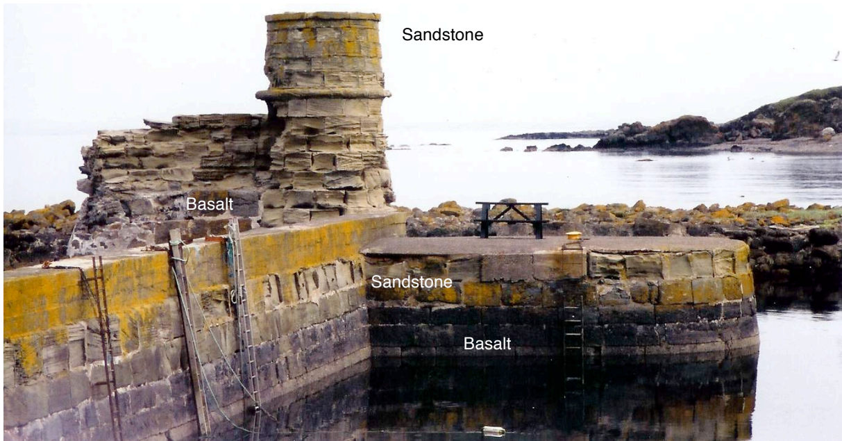
Fig 7: Lighthouse and adjacent harbour walls
